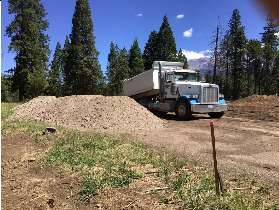
Photo 1: Delivery/import of soil and rock materials
