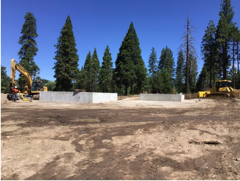
Photo 3: Grading and compaction work within project area
