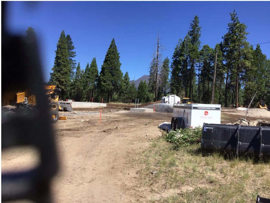
Photo 4: Dust control being implemented (water truck) in accordance with APM AQ-1
