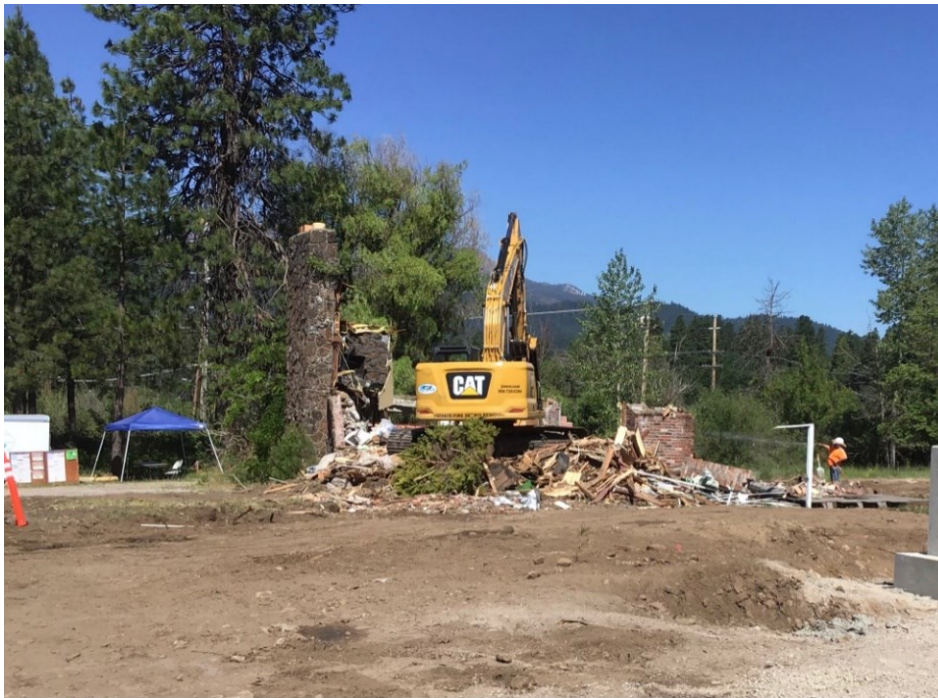
Photo 2: House demolition with dust control being implemented during demolition
